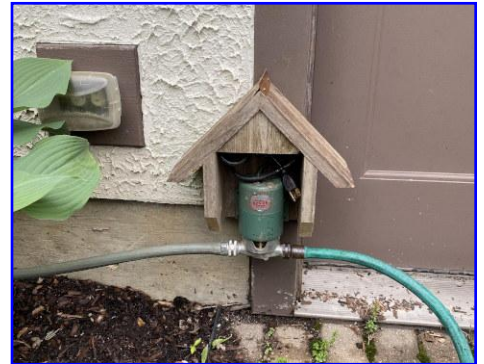
Mike Perry - Pump House for Gardern Hose Cedar, Copper
